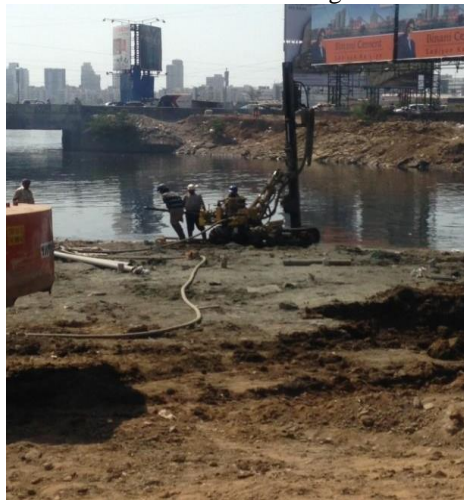
Figure 3. ODEX Drilling at Mithi River near Mahim Bridge
