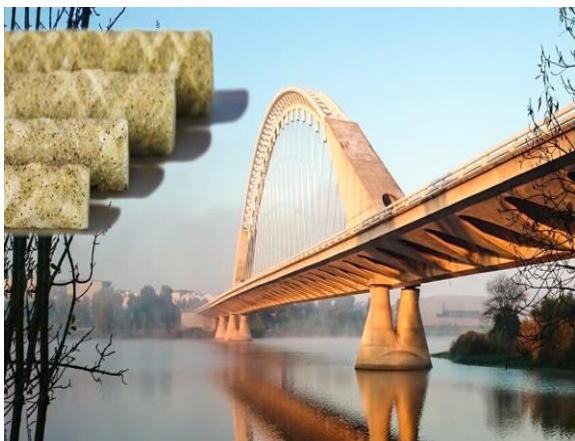
Fig 12: Bridge construction using FRP composite [27]
